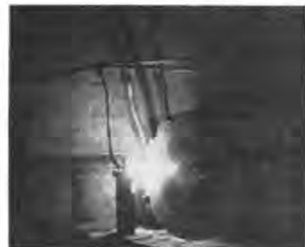
Siasconset's spark. This photograph was made with a 5 sec. exposure while the disc was running at 1800 R. P. M. Although traveling at a speed of more than 100 miles an hour, the studs appear to be standing still, due to the fact that the disc was illuminated only at the instant when the moving stud came opposite the stationary stud, causing the spark to discharge.
